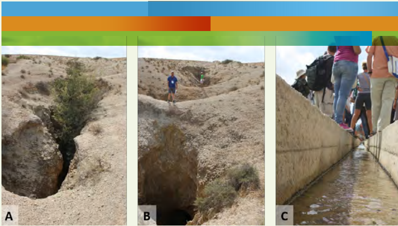
Figure 1 Example of khetaras from the reservoirs of Western Haouz, Morocco (pictures by Eric Rosa)
